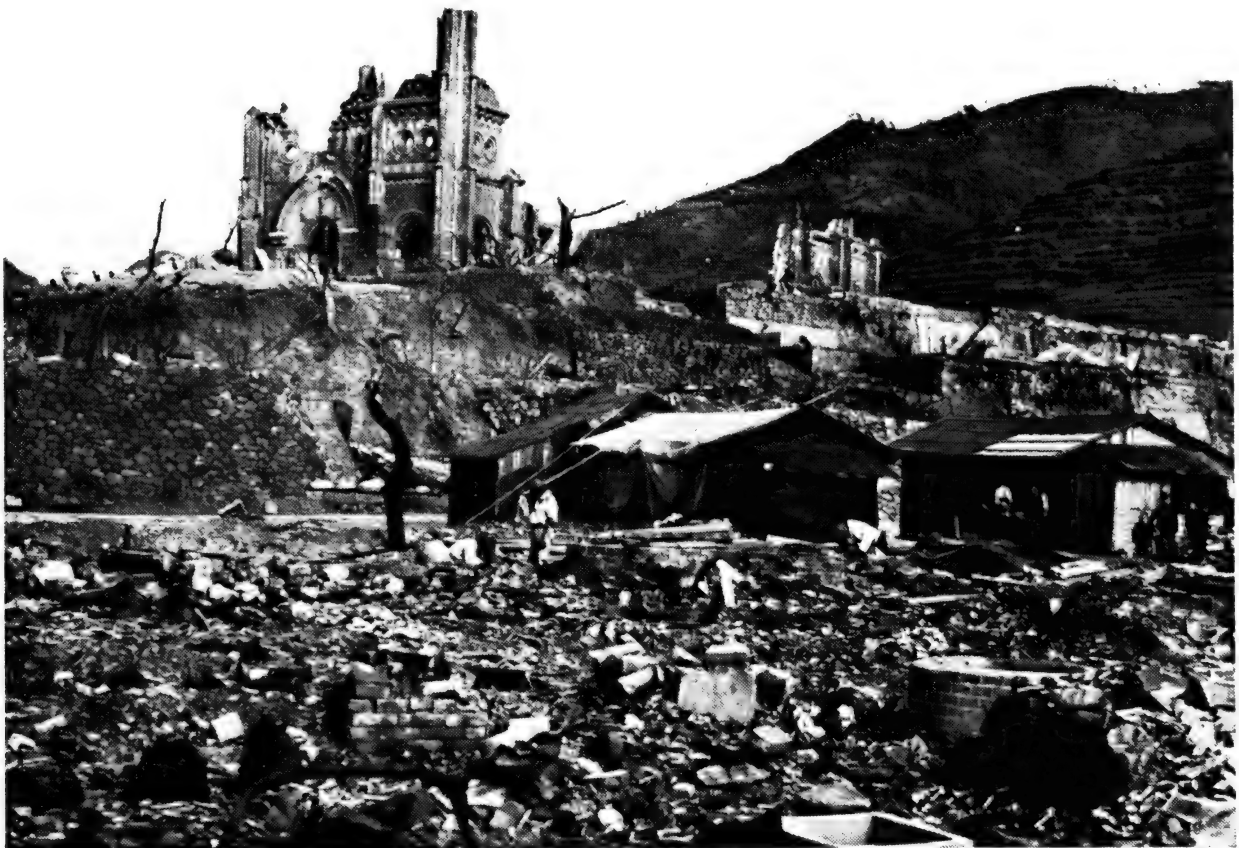
Photo No. 16. NAGASAKI. The Roman Catholic Cathedral 600 yds. from centre of damage. The walls were of heavy load-bearing brick construction. Most of the damage is attributable to blast, although fire subsequently consumed all combustible debris. Note in the foreground the huts erected by the Japanese for temporary living quarters after the atomic bomb raid. See paragraphs 11, 16 and 39.
